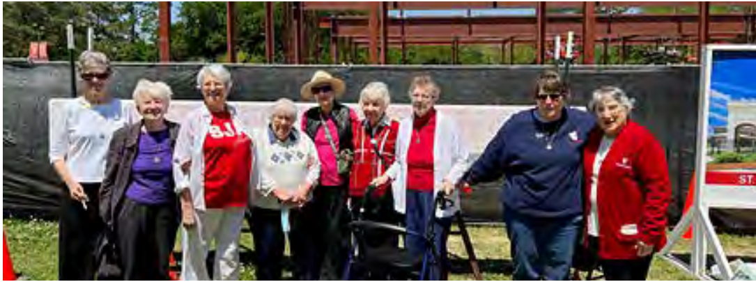
Sisters were invited to come sign the beam which will be installed in the new Student Commons building, currently under construction. Seen above, left to right: Sr. Joan Laplace, Sr. Lucy Silvio, Sr. Dianne Fanguy, Sr. Anna Schellhaus, Sr. CynthiaSabathier, Sr. Evelyn Mee, Sr. Frances Landry, Sr. Chris Pologa and Sr. Adele Lambert
